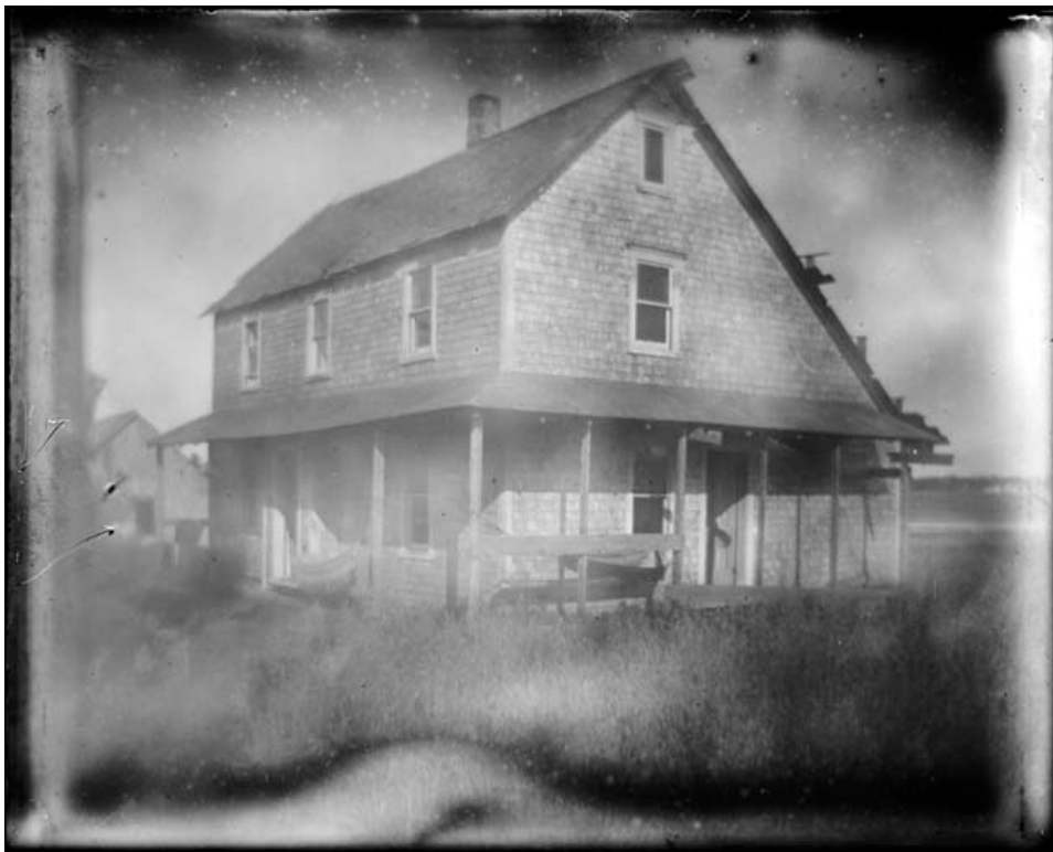
House under construction or repair, rural Prince Edward Island, ca. 1905-1920. Mille Gamble, creator. Public Archives and Records Office of PEI, Acc3885/37
