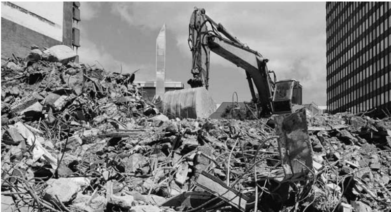
Demolition (DigitalVision stock photo)
